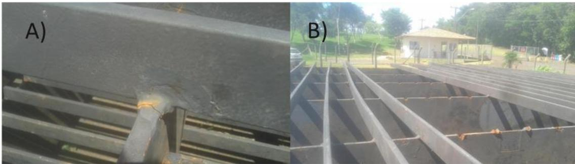
Figure 1. A) Pass-through crack between the front vertical bars and the rack panel tray; B) Failure caused by cracks, with subsequent removal of the vertical bars.
